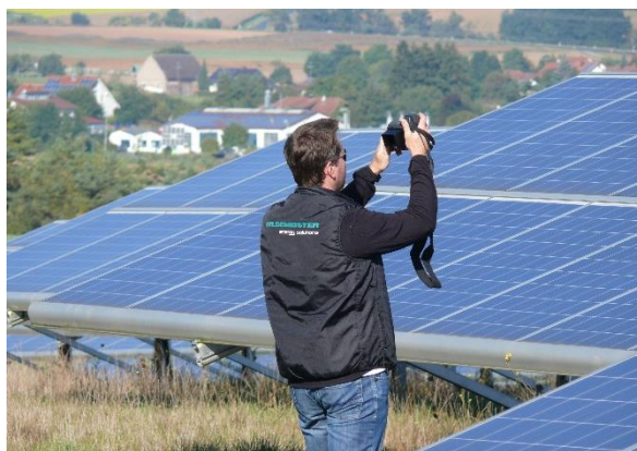
Maintenance des installations photovoltaïques (photo: GILDEMEISTER Energy Solutions GmbH)
