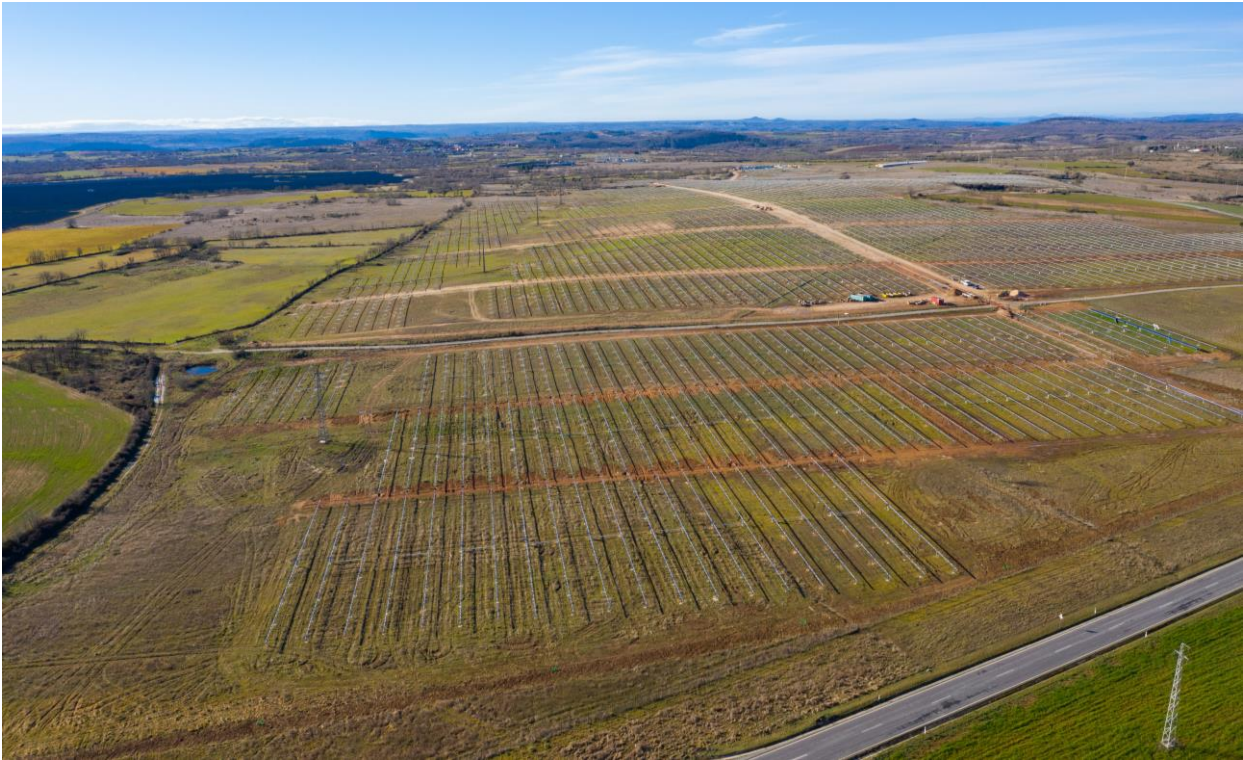
The Betty plant under construction, the Mogadouro plant can be seen in the top left background.
