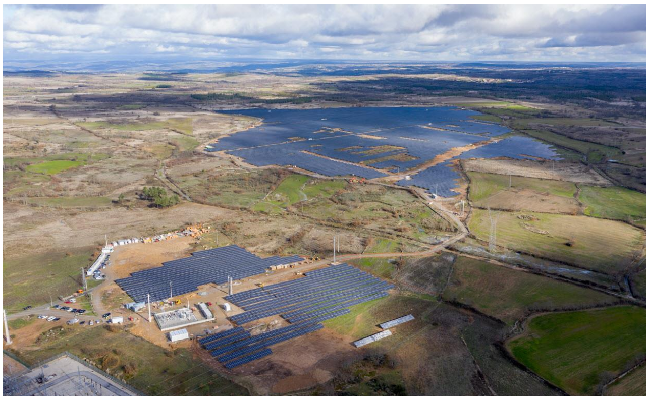
Mogadouro large-scale PV system with space for battery or electrolyzer
