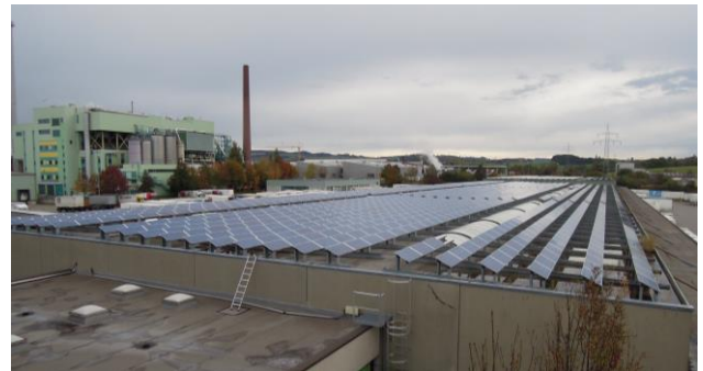
Oldest German PV plant of Edisun Power: Lebert Kempten
